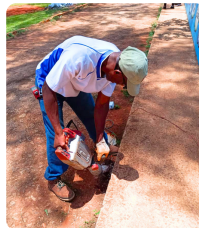
A volunteer working on the walkway.
