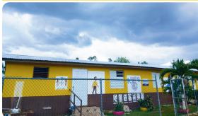
Roof rehabilitation works have been completed at Evergreen Basic School
