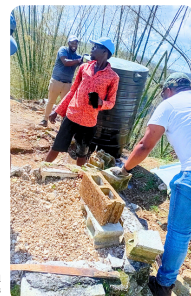
Members of the Jamaica team works to repair Shadeika's grandmother's house.
