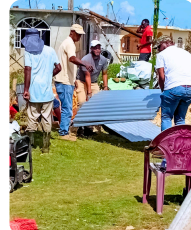
Zinc sheets being moved by members of the Jamaica's team.
